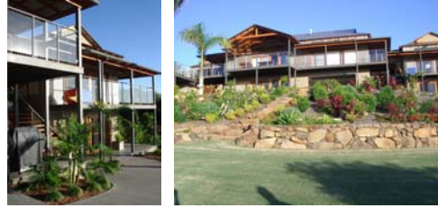
Residence Phoenix Drive, Tintenbar
